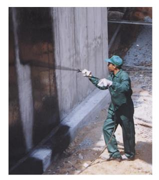
When we set out to define the cases where these sprayed or applied systems should be preferred over using torched bitumen membranes, we should relate to the following:
